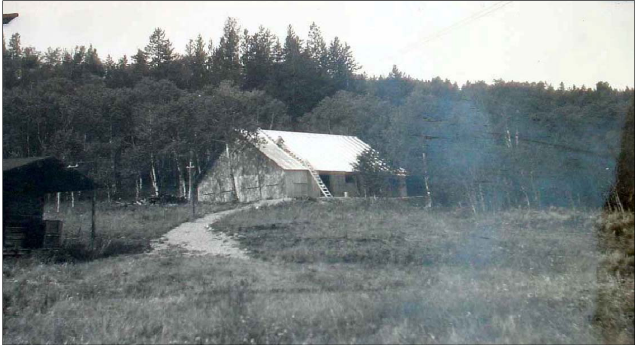
Figure 5: Spray Painting Johnston Hall
